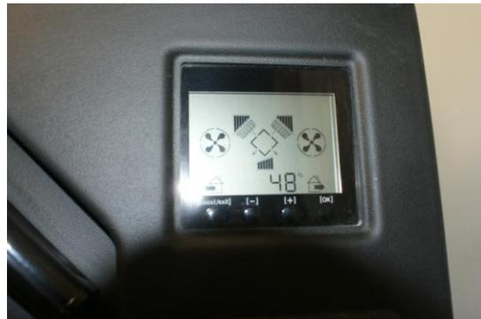
Figure 3: Boost switch and controls on right at top of MVHR Unit
