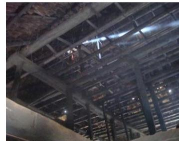
Fig.8. Roof structure mainly from bamboo and covered with dried grass
