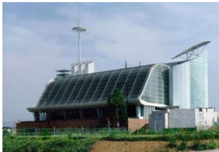
Fig.6. Photograph of the office building
