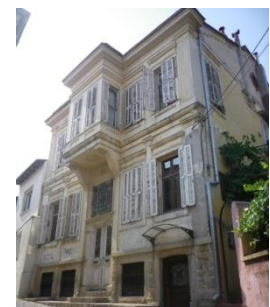
Figure 4. Building of study
