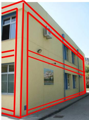
**Fig. 2:** Main cold bridges presentation: structural components.
