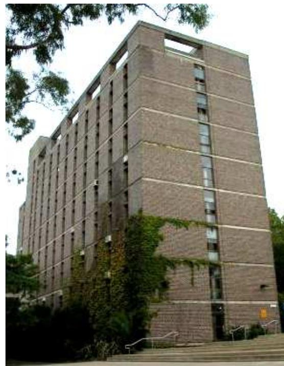
**Photo 2:** MQ, NV building (North façade) featuring occupant-operated windows with some individual air-conditioner units
