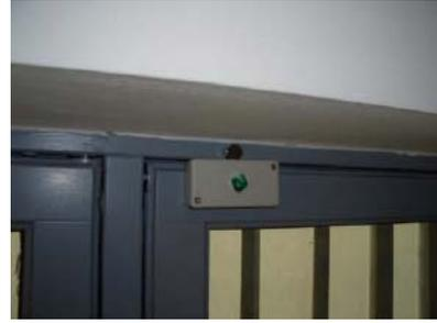
**Fig. 3.** Wireless contact sensor on external door opening
