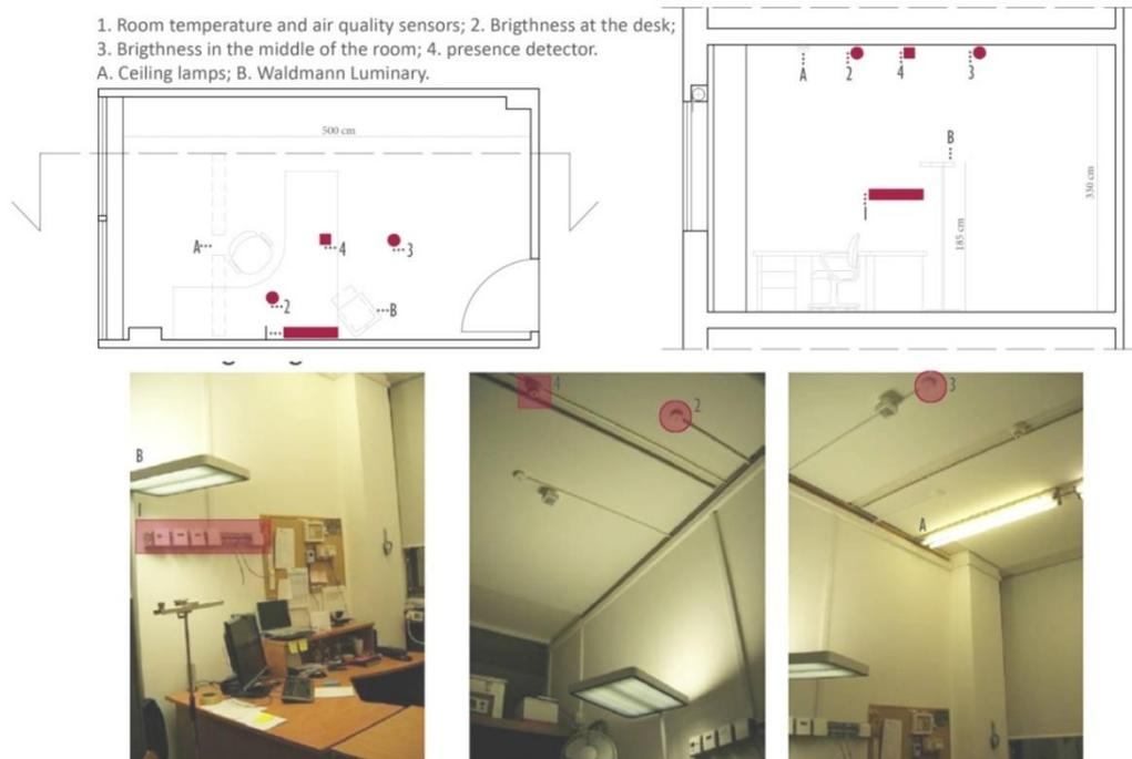
Figure 1. Installed sensors in office rooms.
