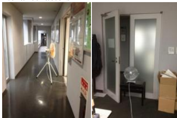
Figure 12. Opening the ventilating doors into the thoroughfare passage ways directly affected privacy; Vertically pivoted windows in the ventilating corridor obstruct free movement of people.
