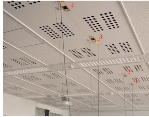
(b) Radiant ceiling panel system and sensors
