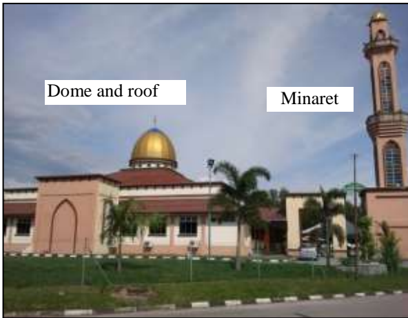
a) Building view from West
